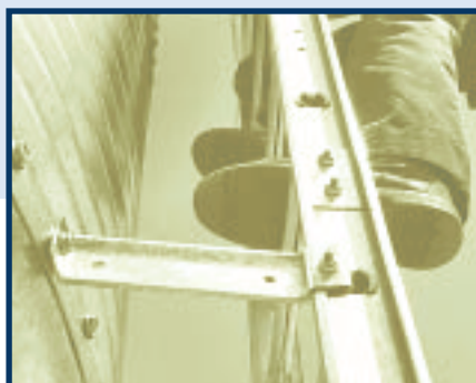
Side ladders allow plenty of space between rungs and bin wall for your feet.
