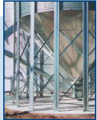
Sturdy "X" bracing between legs gives additional bin strength. Bracing is simple to assemble and offers easy access to boot.
